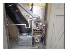
◆ The filter installed in this unit is dirty. This can slow airflow and reduce the efficiency of the system. We suggest cleaning or replacing this filter periodically as part of routine maintenance.
