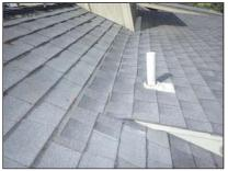
Common moss growth noted which can accelerate the deterioration of roofing materials.
