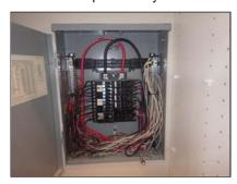
▶ Doubled-up circuitry noted at neutral bar (i.e. 2 neutral wires on a single terminal). This condition can cause wiring to become loose, leading to arcing and overheating. Each grounded conductor should terminate within the panel board in an individual terminal that is not also used for another conductor. We recommend review by a qualified professional electrician for correction, as necessary, to ensure proper operation and safety.
