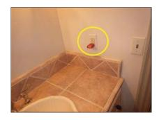
◆ The wall light fixture over the shower did not operate at the time of inspection, possibly due to a burnt-out bulb. We suggest proper operation of the light fixture be demonstrated with a new bulb or repairs be made, as necessary.
