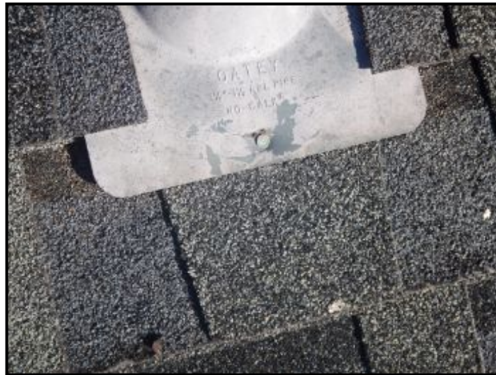
Seal exposed fasteners as needed.
