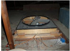
combustion exhaust gases out through the flue pipe, any negative air pressure within the interior of the house could force the exhaust gases back down the flue pipe and into the interior. This fan should only be operated with sufficient open windows to prevent any exterior/interior pressure differential. As this essentially represents an opening in the attic, it will reduce the efficiency of the house during the winter months.
