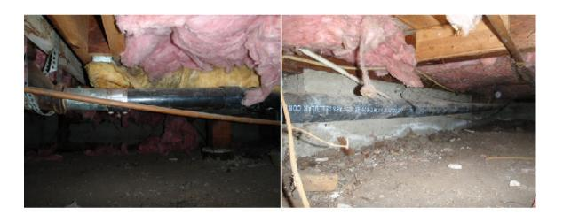
Where visible, waste lines are cast iron, galvanized and ABS (plastic). Older metal waste lines are more likely to be corroded and become clogged than other materials. Client is advised that slow drains and leaks are likely to develop over time due to the type and age of the material.
