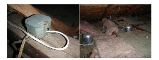
**Unprotected electrical splices present**. Electrical splices should be enclosed in a covered junction box to help prevent separation of the splices.
