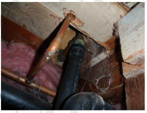
**Openings were found in the subfloor sheathing.** These openings can allow rodents access into areas under bathtubs and into wall cavities. While not required at time of original construction, I suggest screening any openings with a metal mesh.
