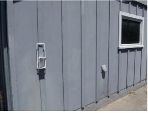
defective siding was found at time of inspection, this general type of product can be more susceptible to swelling due to moisture intrusion than solid wood siding; even with a non-defective product. As such, it is important to keep the exterior of the home, particularly the edges and cut seams of siding and trim, well sealed with paint and caulking to prevent moisture damage.
