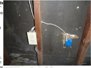
**Receptacle outlets are the older, two pin, non-grounded type.** When grounding is not available, installation of GFCI (ground fault circuit interrupter) devices is advised.
