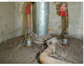
the flue pipe from becoming disconnected. As this cannot be effectively done with this older flue pipe material, replacement is advised. If client has concerns regarding the asbestos material, a testing laboratory should be consulted.
