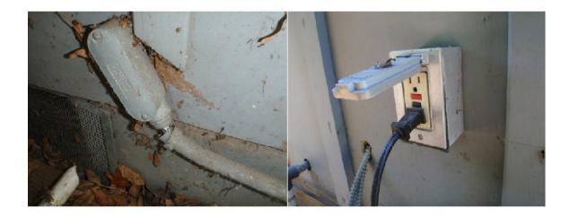
A disconnected conduit was found at the right side adjacent to the water heater closet. The conductors are exposed. This should be reconnected/repaired.
