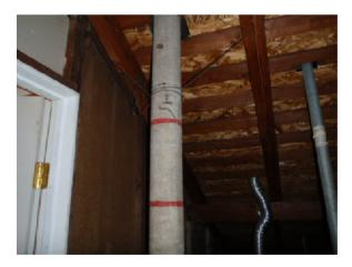
**Flue pipe is improper and damaged.** In addition, the flue pipe in the attic is a "transite" material. I recommend replacement of both sections of flue pipe with a new, metal "bvent" flue pipe.
