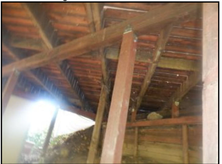
New deck framing installed.
