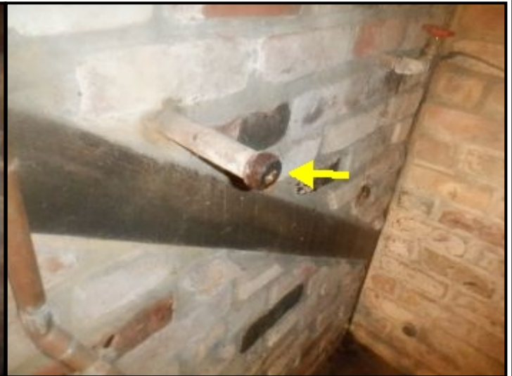
Old leaking plumbing removed.
