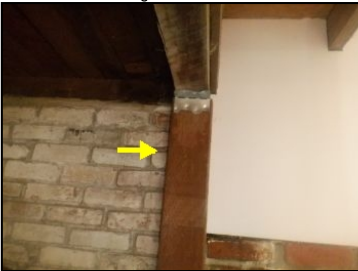
Damaged posts replaced under granny unit.
