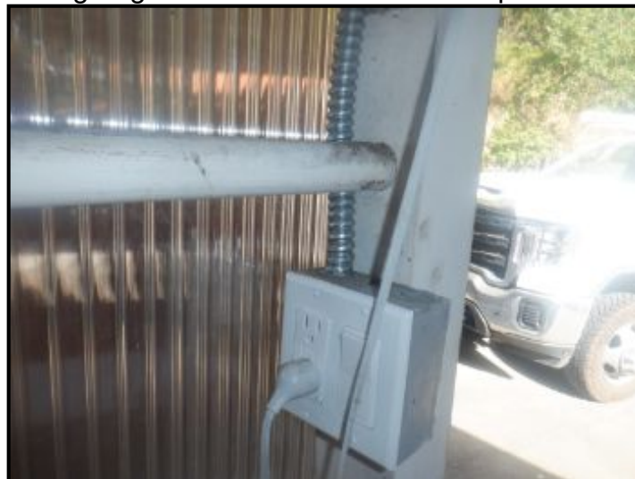
Conduit installed at exposed electrical.
