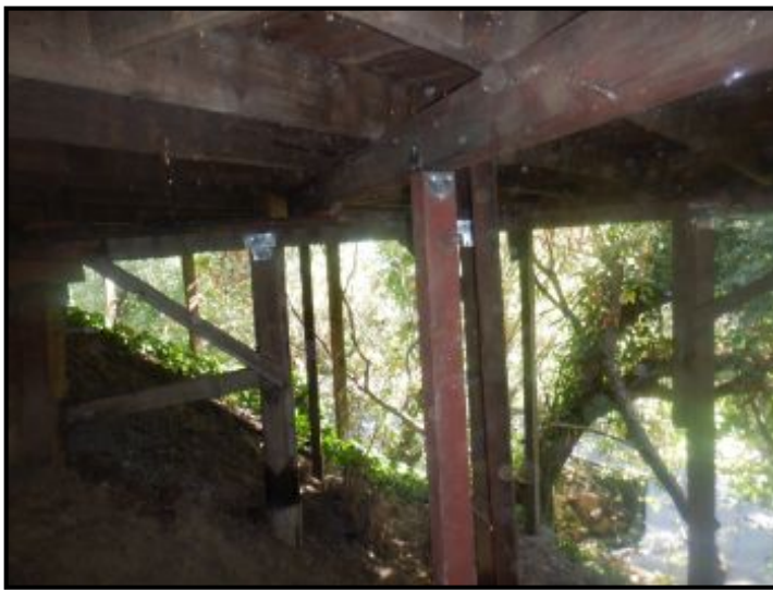
New deck framing installed.
