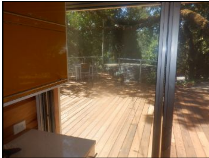
Lost seal at glass slider.
