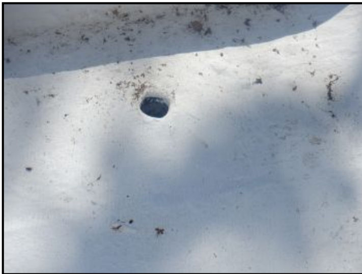
Install screens at drains to prevent blockage.
