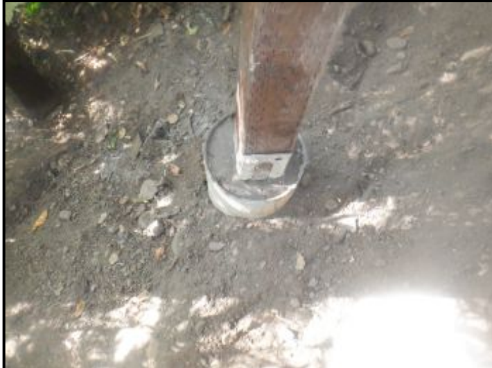
New deck framing installed.
