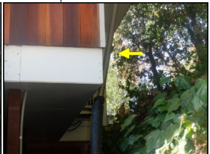
Downspout secured to structure.
