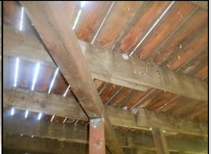
New deck framing installed.
