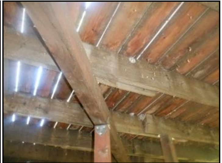
New deck framing installed.
