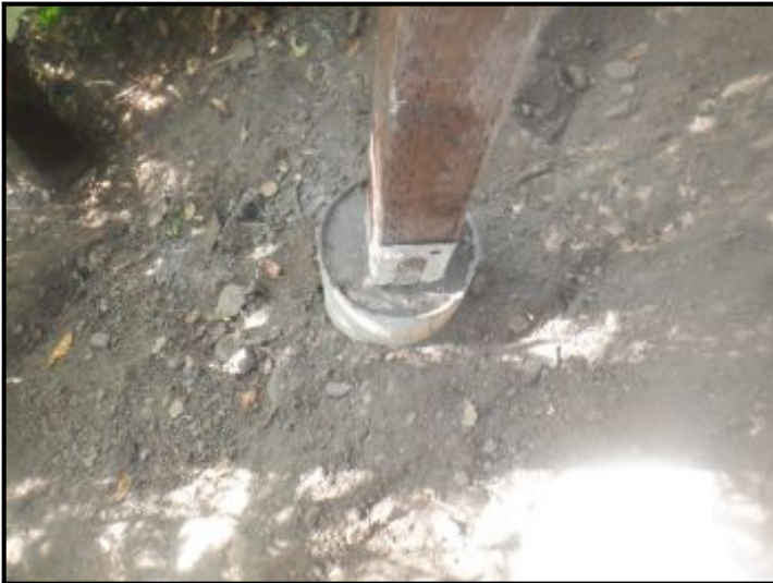
New deck framing installed.
