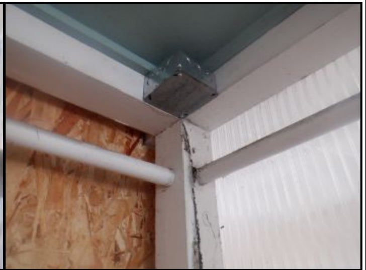
Exposed electrical removed.
