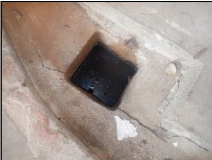
Drain installed at right side of home.
