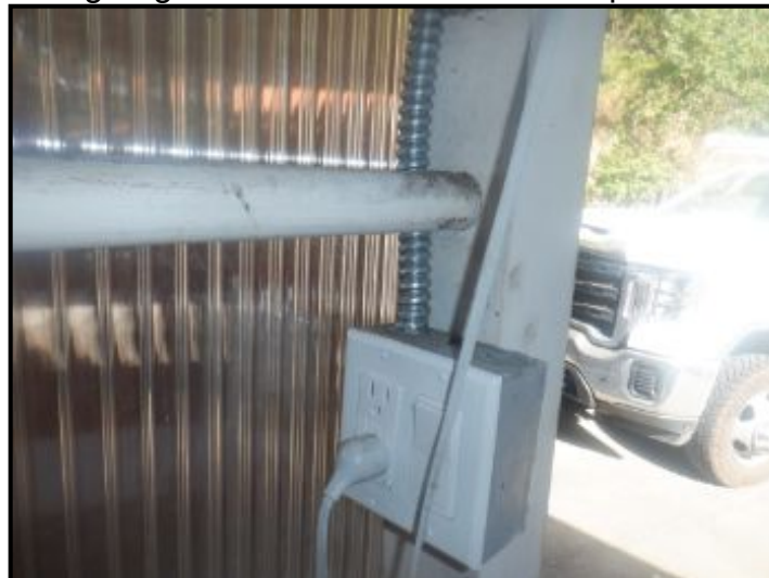
Conduit installed at exposed electrical.
