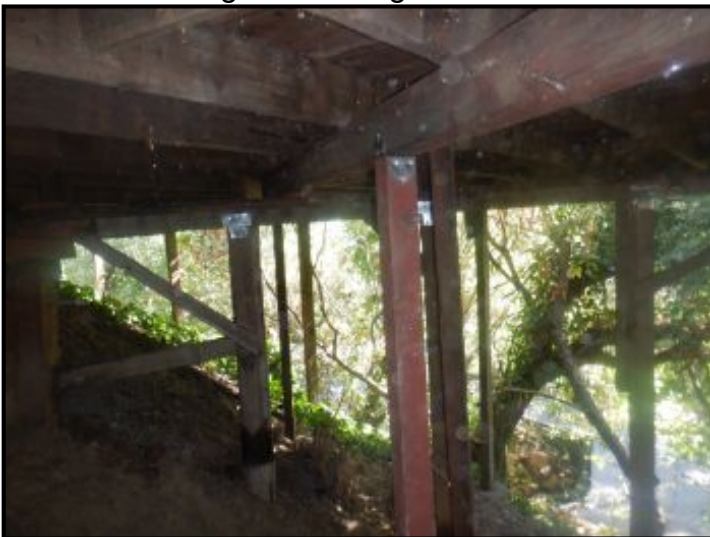
New deck framing installed.
