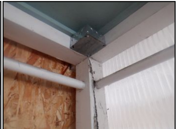
Exposed electrical removed.
