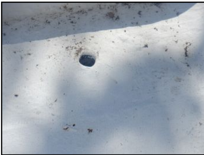
Install screens at drains to prevent blockage.
