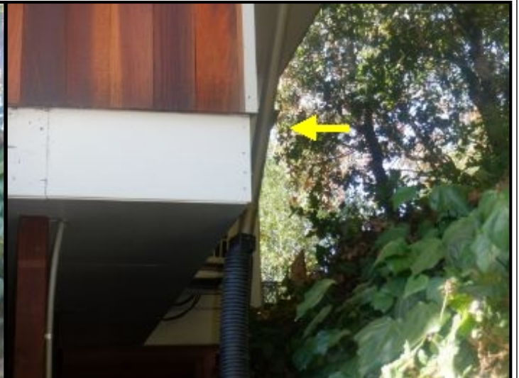
Downspout secured to structure.
