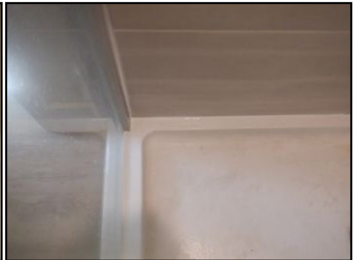
New caulking installed at granny unit shower.
