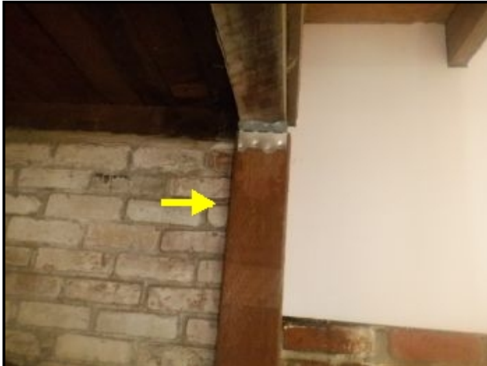
Damaged posts replaced under granny unit.
