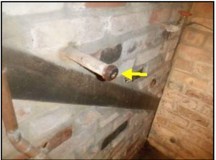
Old leaking plumbing removed.
