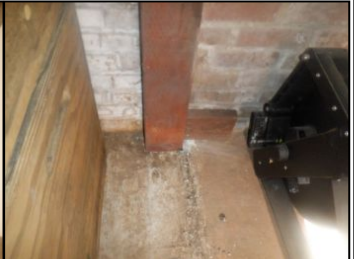
Damaged wood members replaced under granny unit.
