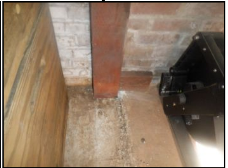
Damaged wood members replaced under granny unit.
