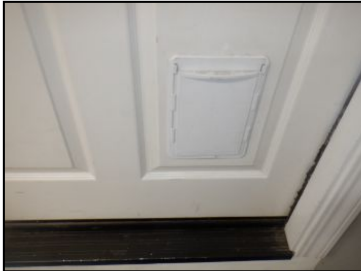
Pet door installed at garage door.
